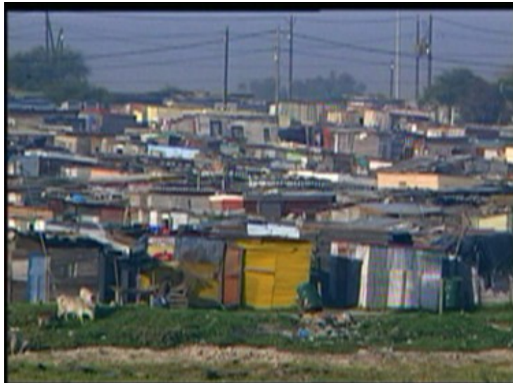
Figure 1.? Electricity supply to informal settlements is often shared illegally among neighbors or siphoned off the main supply.
